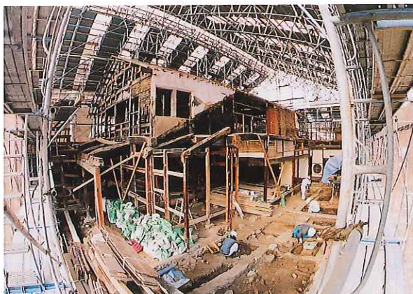
Restoration and repair work
